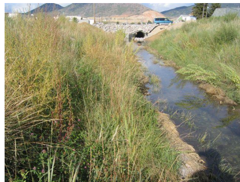
Figure 8. Established vegetation on the reclaimed Metro Storm Drain, along with the meandering pilot channel to “renaturalize” the MSD.
