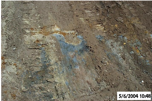
Figure 5: Removal of Visible Mine Waste.
