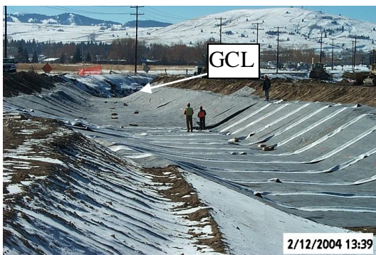
Figure 7. Construction of the Metro Storm Drain Channel.
