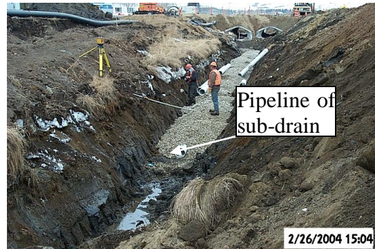
Figure 6. Metro Storm Drain Sub-Drain.
