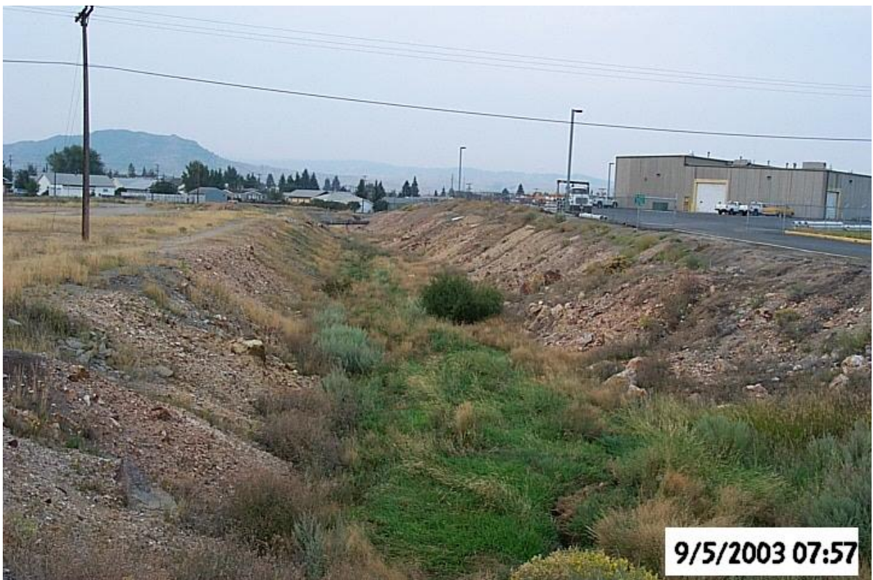
Figure 2. Metro Storm Drain Channel (Pre-reclamation).
