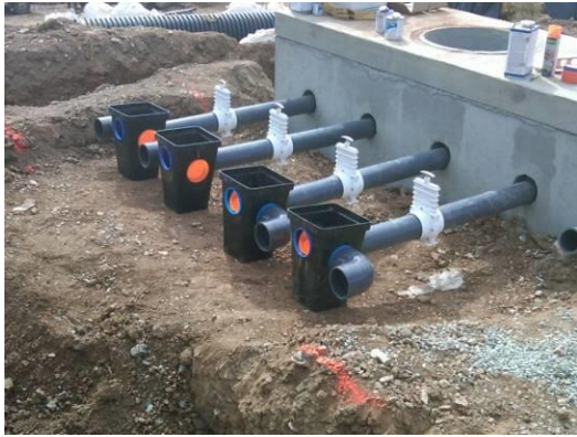
Figure 4. Flow splitter boxes and concrete distribution vault during construction
