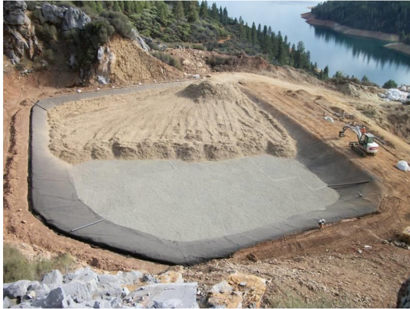
Figure 7. Filling BCR with organic substrate
