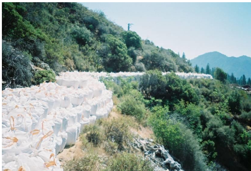
Figure 6. Stockpiled supersacks of construction materials
