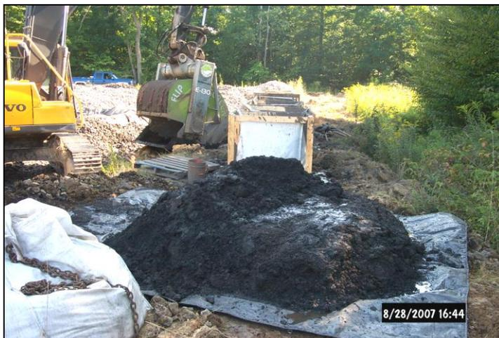
Figure 6. View of recovered manganese material excavated from wash pit
