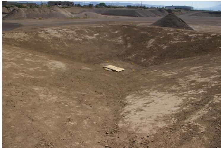
Photo 1. Inside of pilot cell with berms prior to liner placement.
