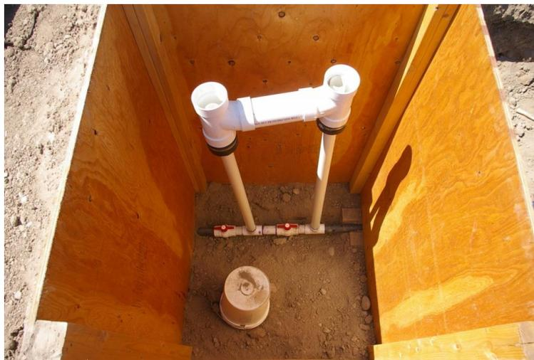
Photo 3. Effluent water level control structure.
